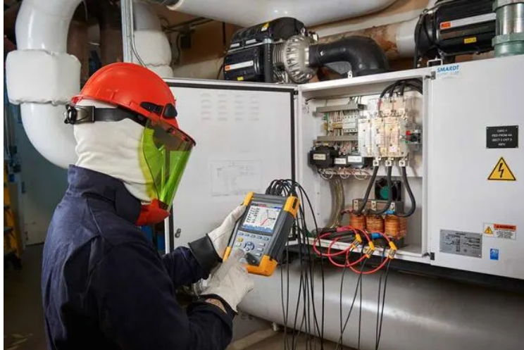
Field measurement and analysis of energy use across electrical, thermal and mechanical systems, carried out to international standards
